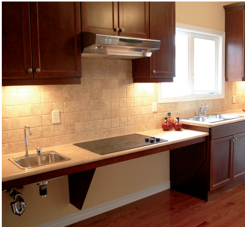
Wheelchair accessible kitchen
